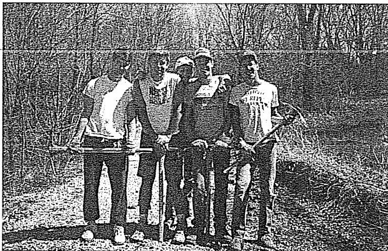
Building the road, early 1960s
